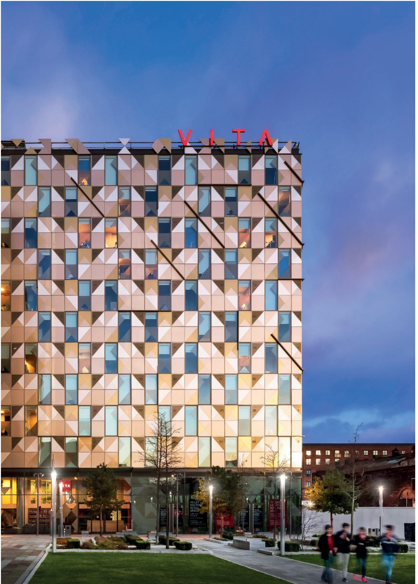
Manchester, First Street
